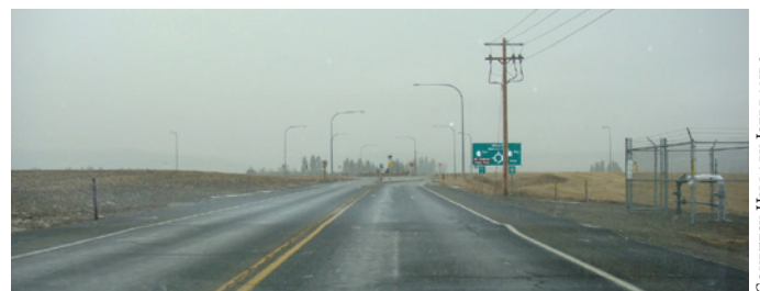
SR 206/Bruce Rd Intersection, 2005 Roundabout Construction, Washington State.
