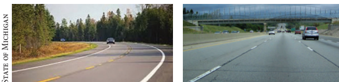
Figure 4. Left: Two-way, two-direction roadway with a yellow skip marking. Right: a multi-freeway with white skip lane marking.
