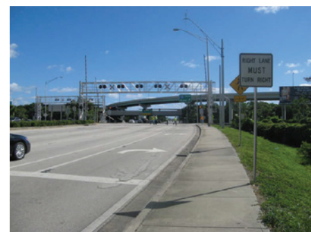
b. Misleading pavement markings and signage.
