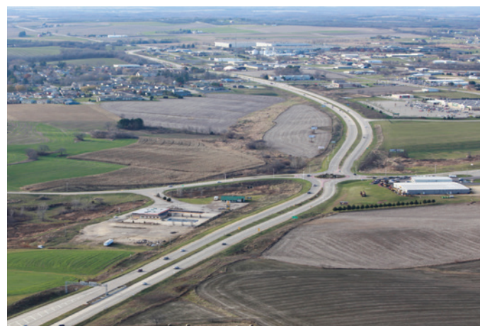
Figure 4. Divided highway in Dodgeville, WI US Hwy 18 at Bennett Rd Intersection.
