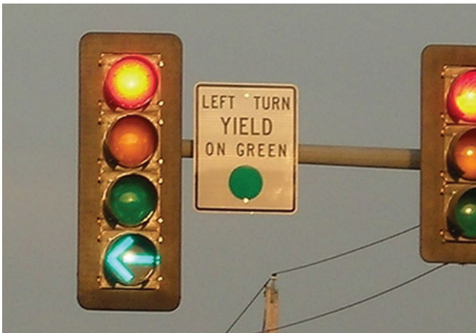
Figure 6. Four-section signal head with green indication.
