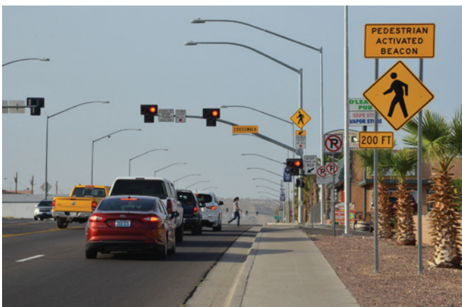
Figure 1. Example of a pedestrian hybrid beacon on SR 95 at 5th Street in Bullhead City, AZ, USA.
