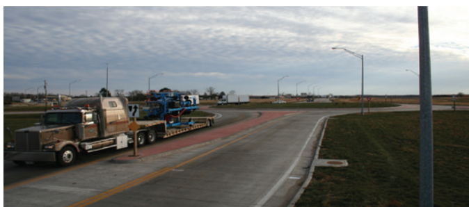
A 2006 Florence, KS, USA rural roundabout US 50/US 77 with a 160 ft.-long splitter island.
