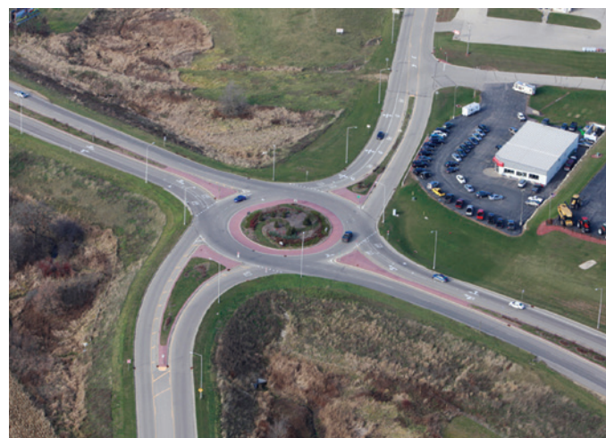
Figure 2. USH 18 at Bennett Road Dodgeville WI, USA.
